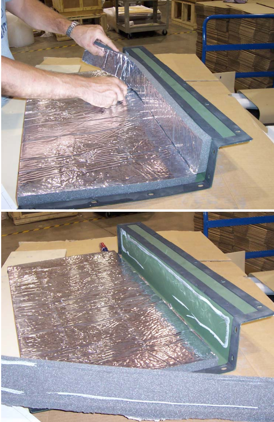
Figure 3-70. Doghouse Insulation Modification.
